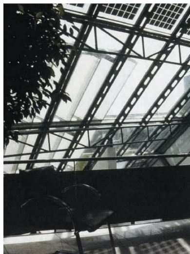
Fig. 15. Glass transparent envelope with holographic film
