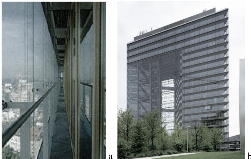
Figs 12 a,b: The building of 'Düsseldorf city gate', Germany, 1999 Architect: Petzinka, exterior view (a), cavity view (b) (Source :H.Poirazis 2004)
